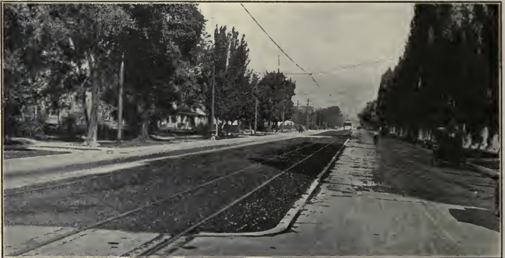
VIEW ALONG 7TH EAST STREET, SHOWING NEW PARK AREA FORMED BY MOVING STREET RAILWAY TRACKS
